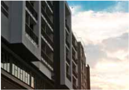
Bedford Square Residential Building, Murray & Roberts Construction Johannesburg, South Africa
